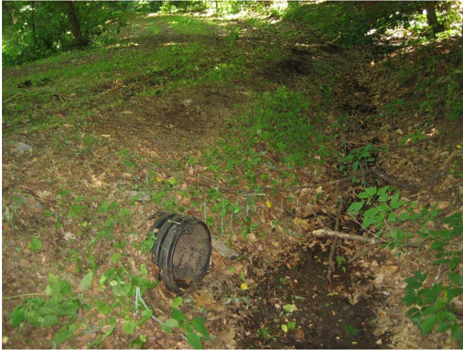
Photo 71: Corrugated plastic pipe inlet on the Township-owned parcel.
