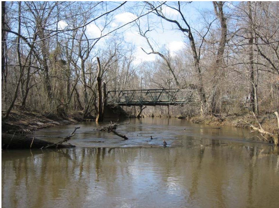
Photo 22: Iron Bridge Road, viewed from upstream, facing downstream (west/southwest).
