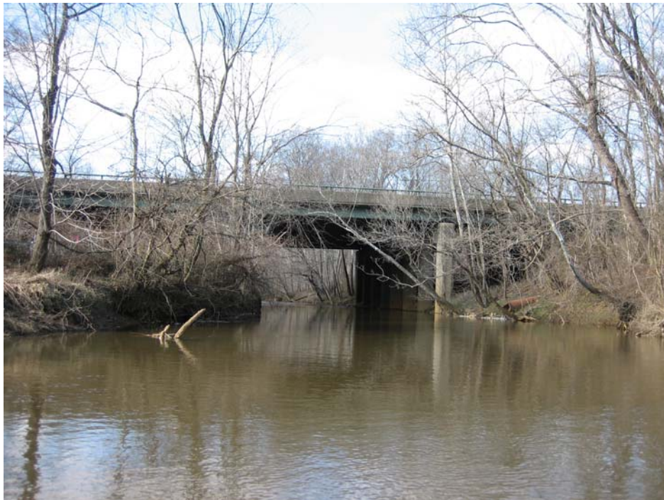
Photo 88: The NJ Turnpike bridge, viewed from upstream, facing downstream (northwest).
