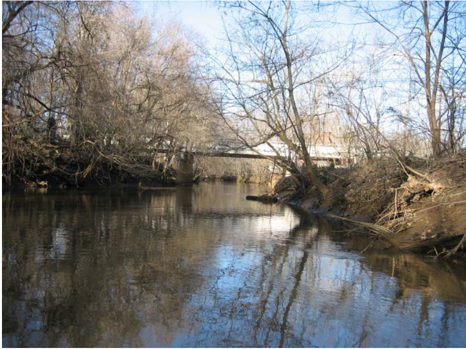
Photo 103: Groveville Road bridge, viewed from Crosswicks Creek, facing downstream (north/northeast).
