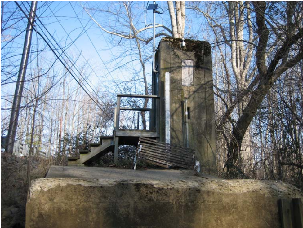
Photo 2: USGS Gaging Station No. 01464500 located at the Extonville Road bridge.
