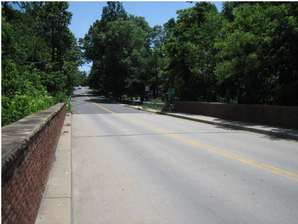
Photo 60: Church Street bridge, facing north (towards Hamilton Township).
