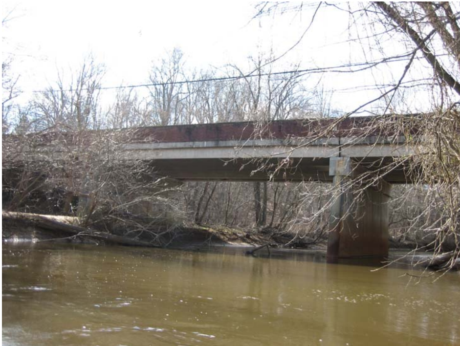
Photo 58: Church Street bridge, facing downstream (southwest).
